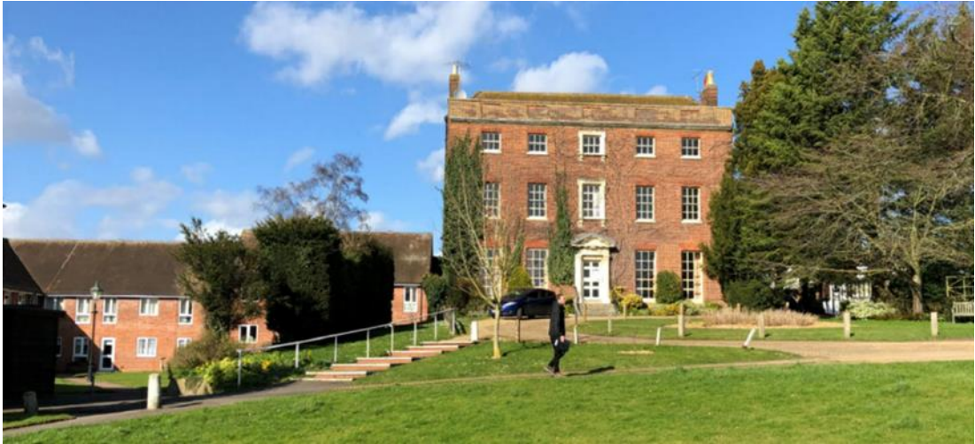
Fig 6b – This shows the relationship of Walden place and the ground level difference
